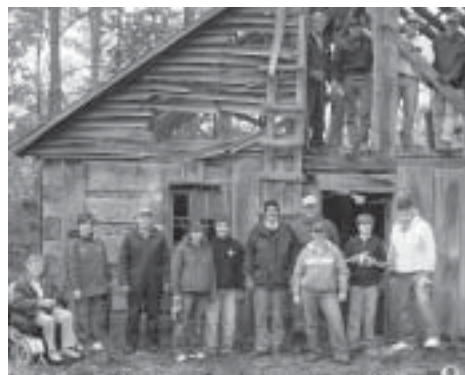
Members of the Tschantz-Schantz family turned out to dismantle the house.
