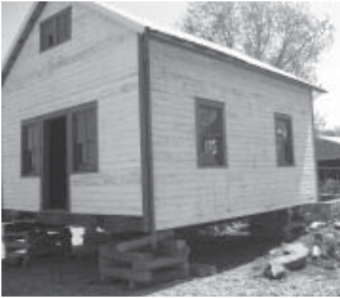
Above: The Lehman Spring House raised up on blocks, next to its original site. Right: Heading up Schneck Hill on Zuercher Road, toward Sonnenberg Village. Below: The spring house arrives at its new home. It is now located to the west of its long-time companion, the Lehman House.
