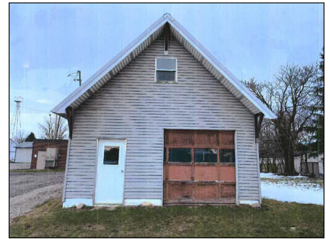
The Moser Buggy Shop has been dismantled and will be reconstructed in the Sonnenberg Village.
